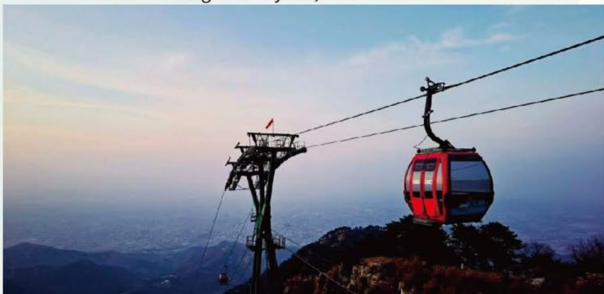
山东泰山中天门索道 Project of Zhongtianmen Ropeway on Mount Tai in Shandong Province
