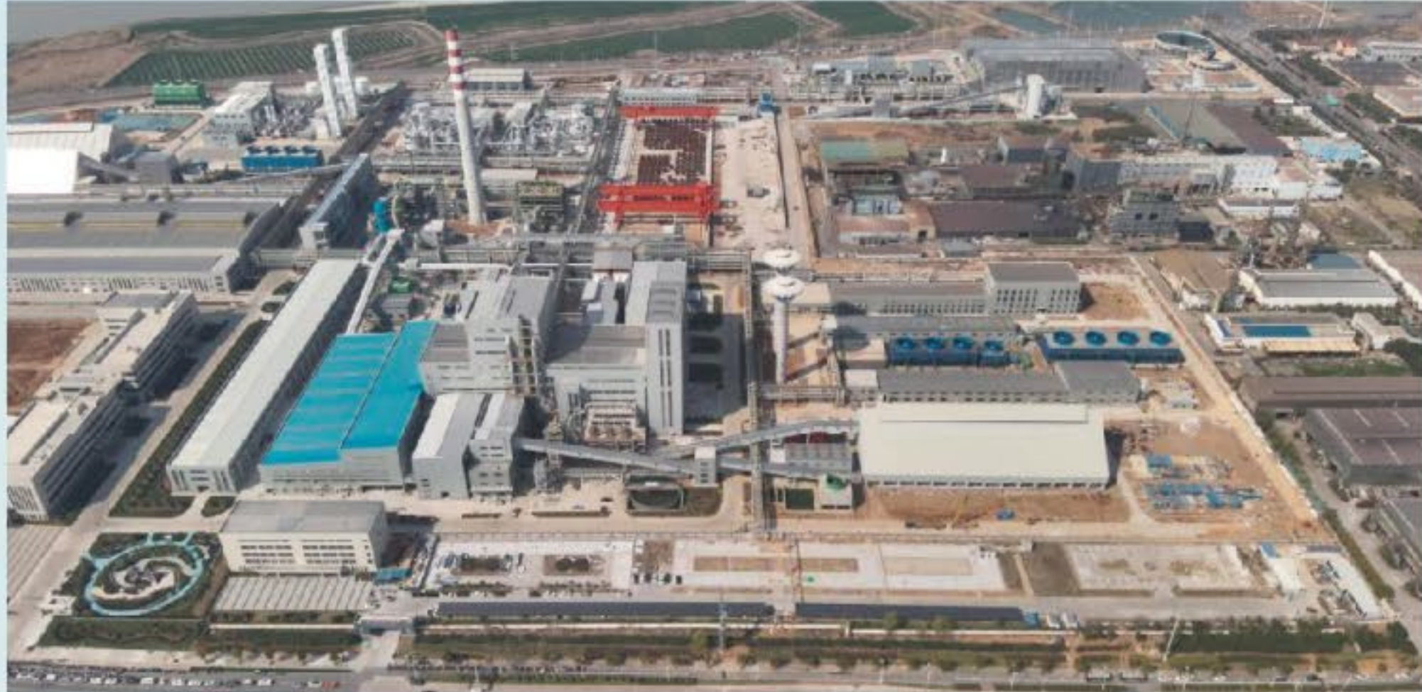
铜陵有色绿色智能铜基新材料项目 Green Intelligent Copper-based New Materials Project of Tongling Nonferrous Metals Group
