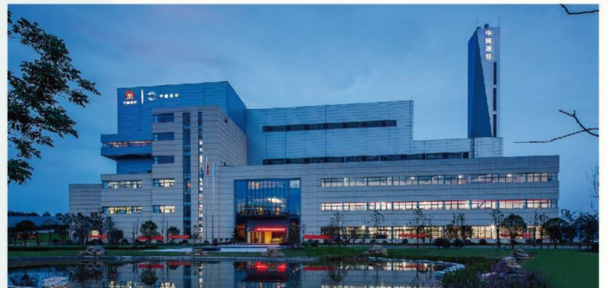
赣州市生活垃圾焚烧发电厂 Project of Domestic Waste Incineration Power Plant in Ganzhou City
