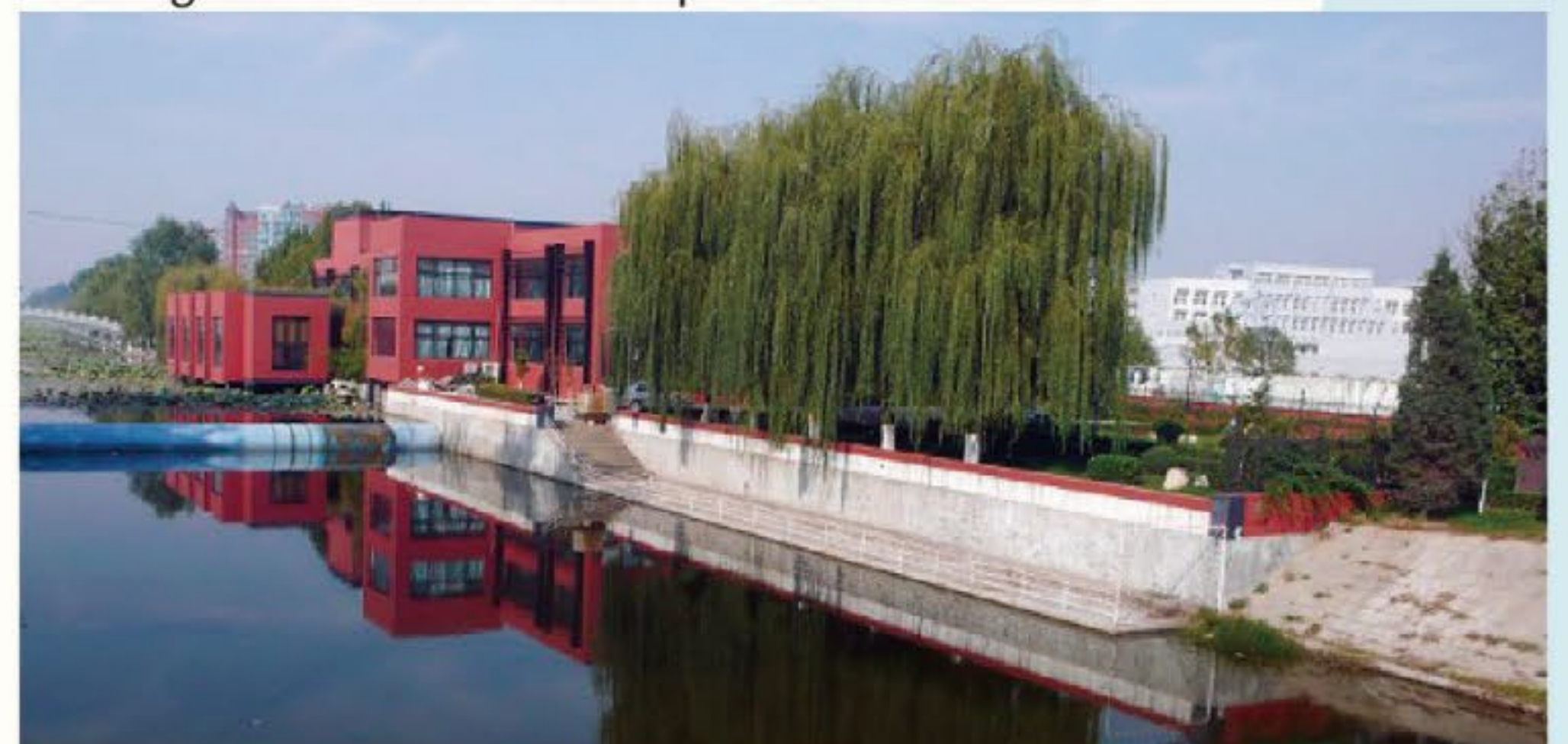
北京良乡污水处理厂 Liangxiang Satellite Village Sewage Treatment Plant
