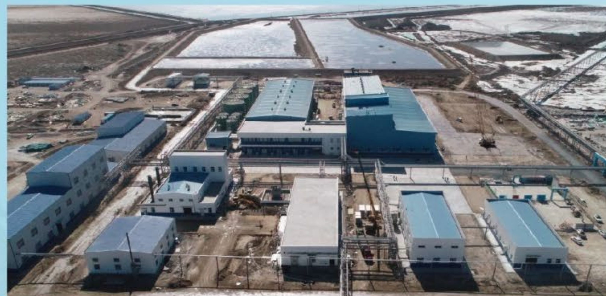
五矿盐湖项目 Project of Salt Lake for China Minmetals Corporation
