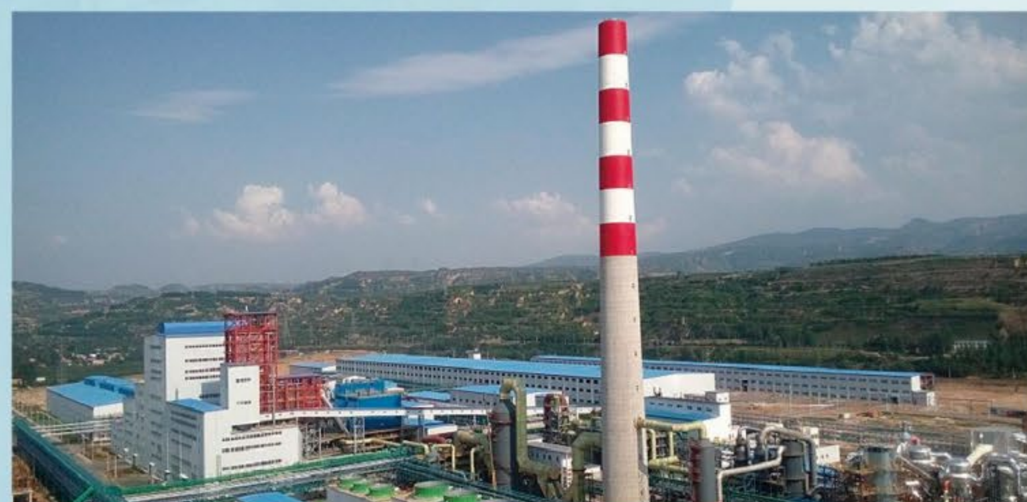
中原黄金项目 Project of Zhongyuan Gold Metallurgical Plant Co., Ltd.
