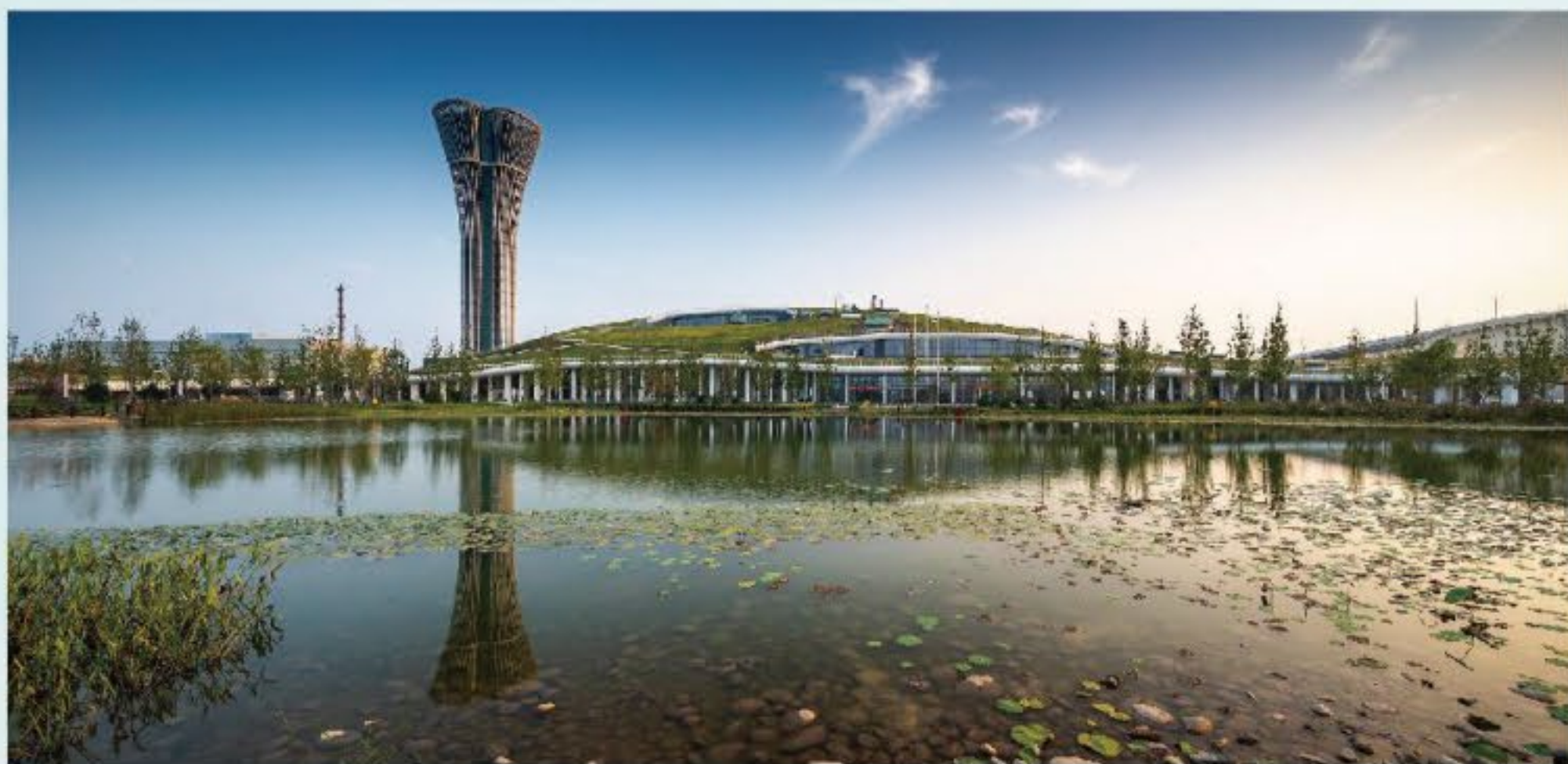
雄安新区垃圾综合处理设施一期工程 Phase I Project of Waste Comprehensive Treatment Facilities in Xiong'an New District
